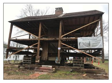
A full building permit has been issued for the project, and the building was handed over to contractor George Fay on April 3, 2017. The building has been lifted and we are now working to stabilize the chimney and create the new foundation. The house will be lowered onto the new foundation and George Fay can begin the next phase of renewal and construction.
