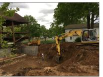
Since April 3, 2017, George Fay has been the project's contractor. The building has been lifted, the chimney stabilized, and the dirt dug out for the new foundation. The next phase is to pour the new foundation's concrete and let it settle. The house will then be
