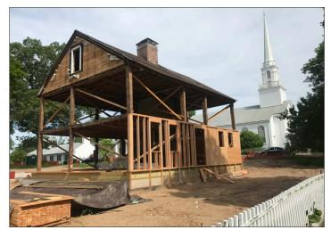
Since April 3, 2017, George Fay has been the project's contractor. The building has been lifted, the chimney stabilized, and the dirt dug out for the new foundation. The concrete for the new foundation was poured and has now settled. George Fay can begin the next phase of renewal and construction.
